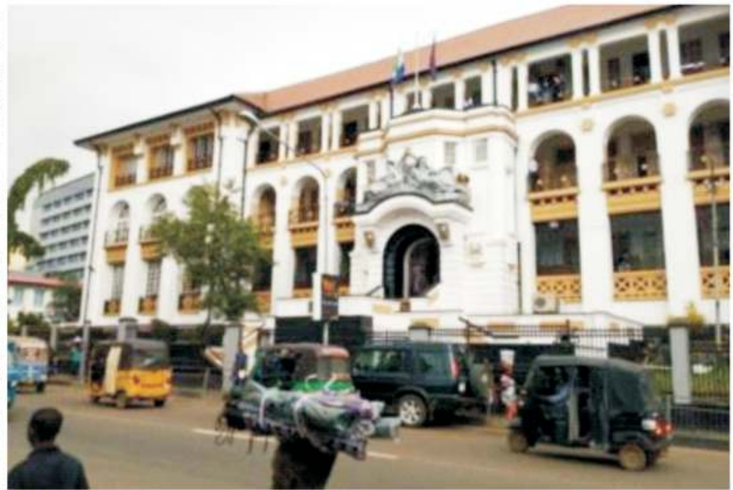
Siaka Steven Street High Court building
